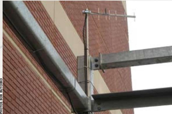
A roof-mounted antenna serves as the anchor point for an in-building public safety radio system.
